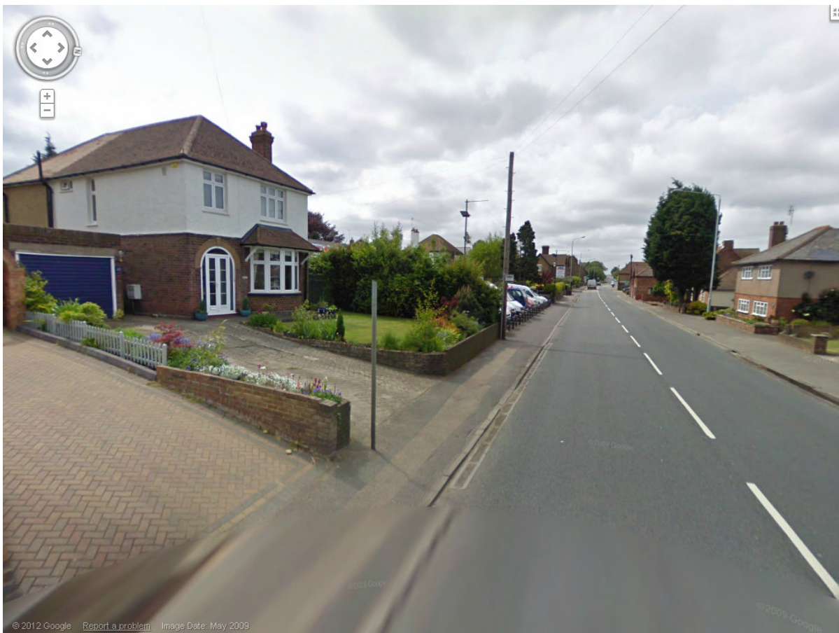
Image: Existing bus stop, looking west towards Sittingbourne
